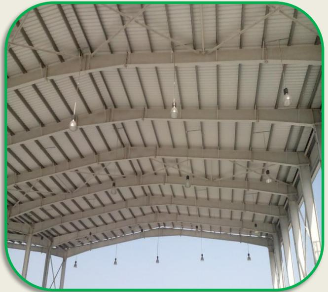
**Steel structure with sandwich panel**
