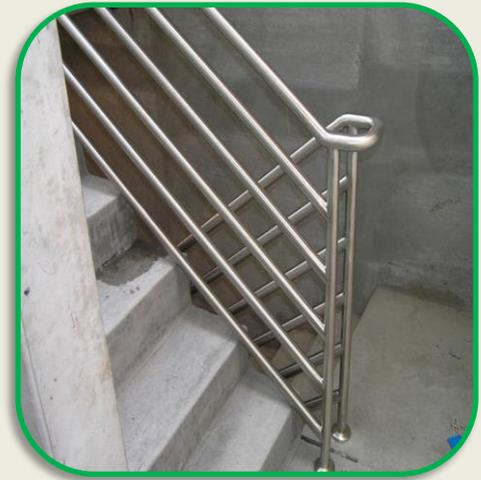
**STAINLESS STEEL HANDRAIL WITH NO MIDDLE BALUSTRADS**
